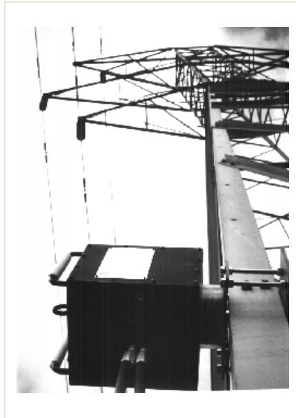
ES-301-2 used for modal excitation of a transmission tower.
